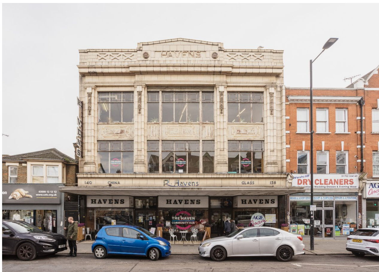
Haven Community Hub, Southend-on-Sea
