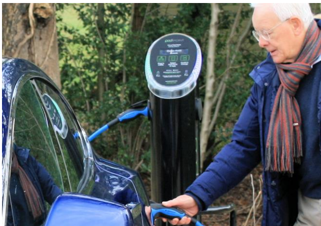
Images: Brighton Energy Coop/Bolney Wine Estate;
